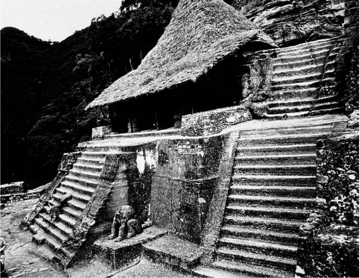
159 Temple I at Malinalco as it is today, with its reconstructed thatched roof.
